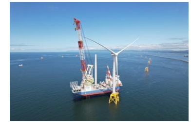
<Turbine Generator Installation>
